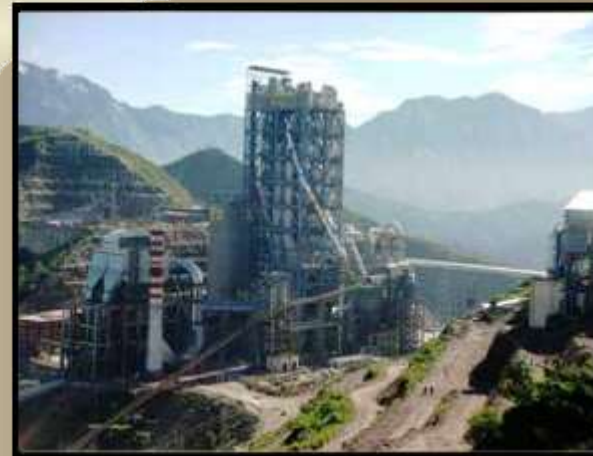
Jaypee Cement, Baga, Himanchal Pradesh, India 10000tpd Cement plant-Preheater tower with composite columns steel structure
