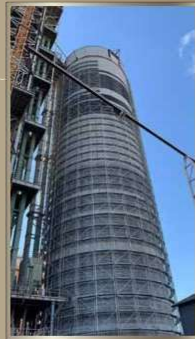
HeidelbergCement-Canakkale, Turkey Repair of disestered Raw meal silo
