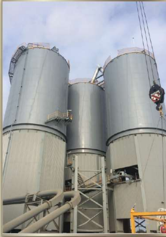
Cement Australia, Osborne, South Australia Remediation of 4X750t steel silos
